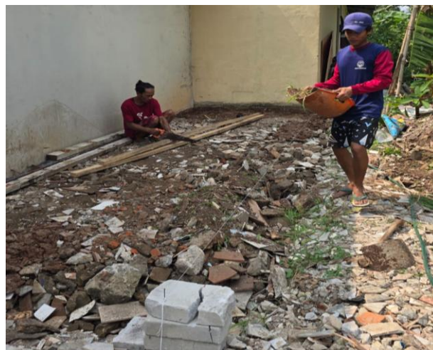
Figure 2. Preparation for Floor Slab Construction
