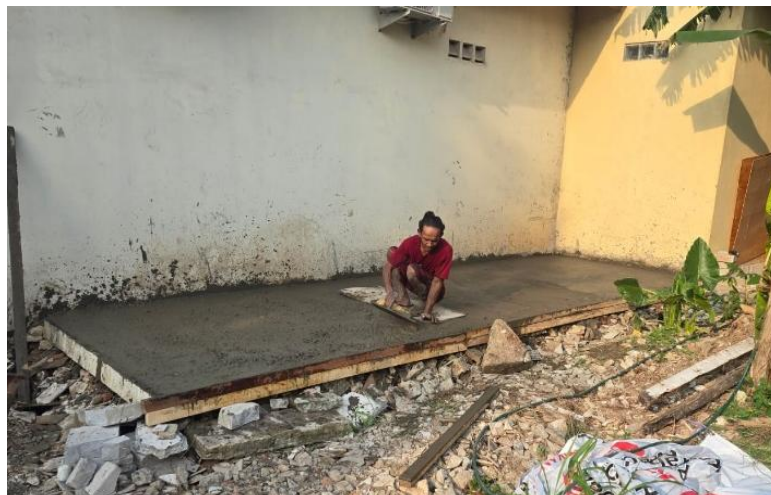
Figure 3. Floor Slab Construction
